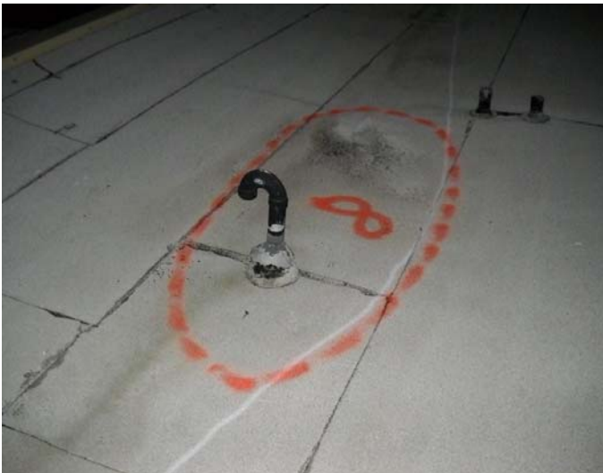
ANOMALY AREA: 8 Date: 8/6/2009 11:55:45 Notes: Suspect area of moisture as indicated.
