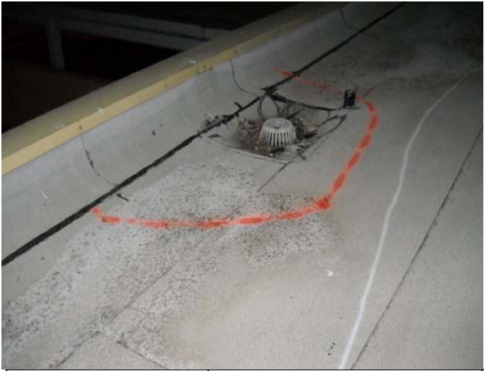
ANOMALY AREA: 5 Date: 8/6/2009 11:16:18 Notes: Suspect area of moisture as indicated.
