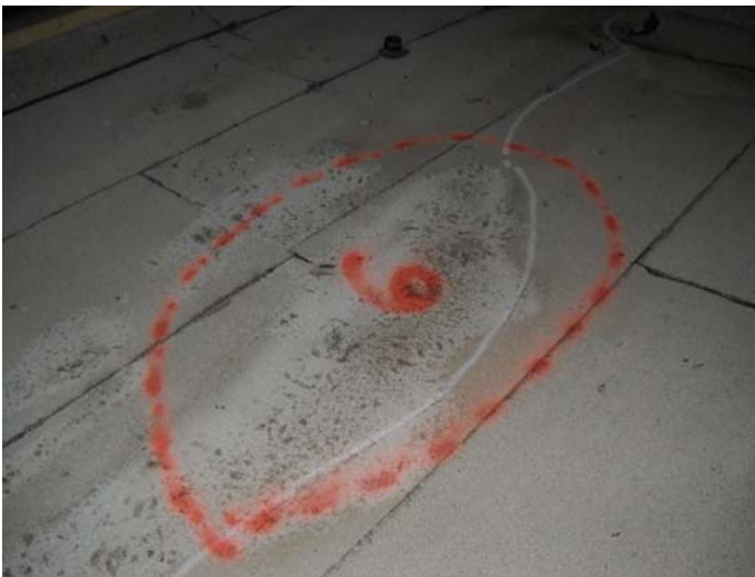
ANOMALY AREA: 6 Date: 8/6/2009 11:21:01 Notes: Suspect area of moisture as indicated.
