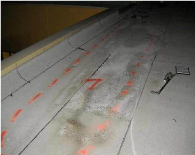
ANOMALY AREA: 7 Date: 8/6/2009 11:39:50 Notes: Suspect area of moisture as indicated.
