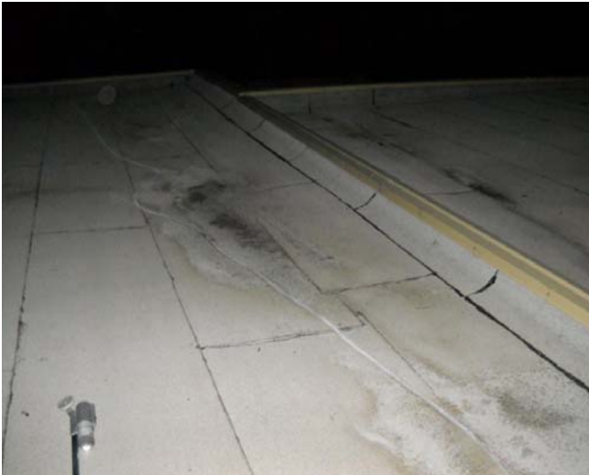
ANOMALY AREA: 1 Date: 8/6/2009 10:40:55 Notes: Suspect area of moisture as indicated.
