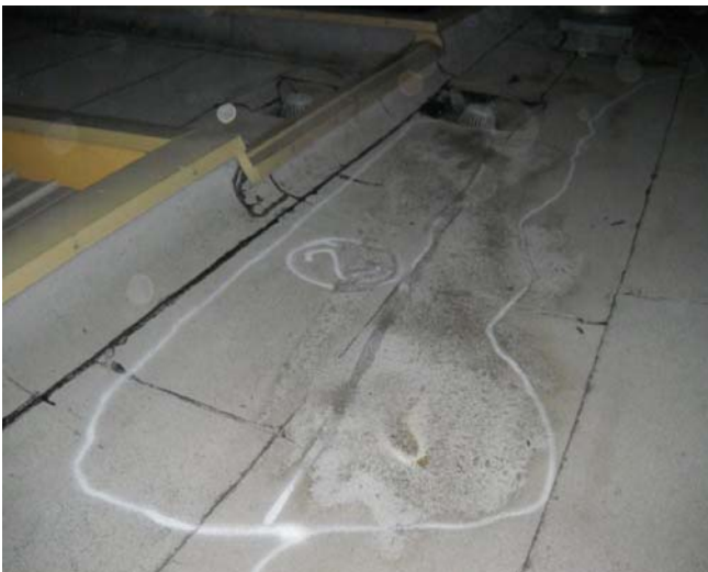
ANOMALY AREA: 2 Date: 8/6/2009 10:55:02 Notes: Suspect area of moisture as indicated.
